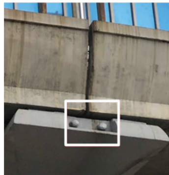
(d) Polymeric coating applied over cementitious caps and exposed to sunlight
