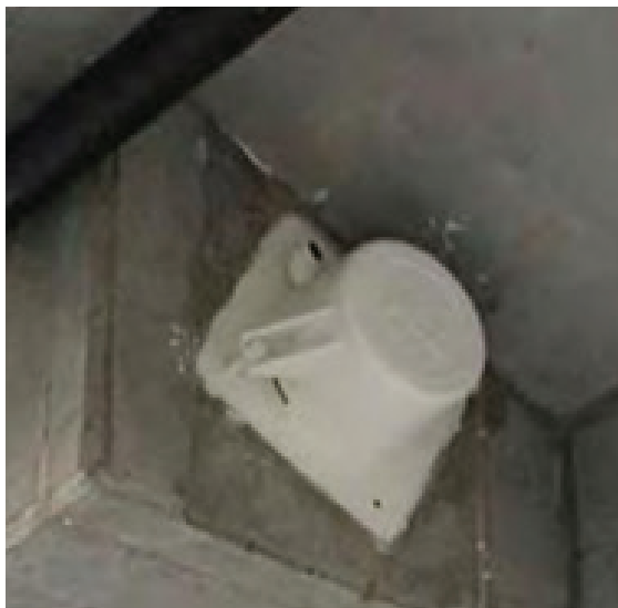
(a) Non-metallic anchorage cap
